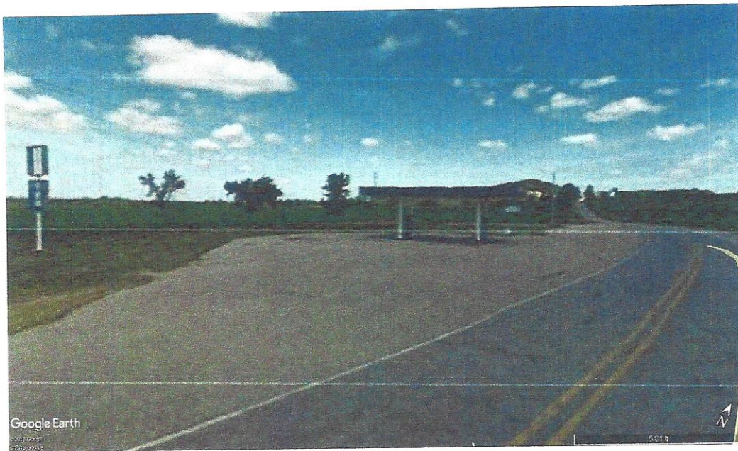
Figure 2 View of the site.
