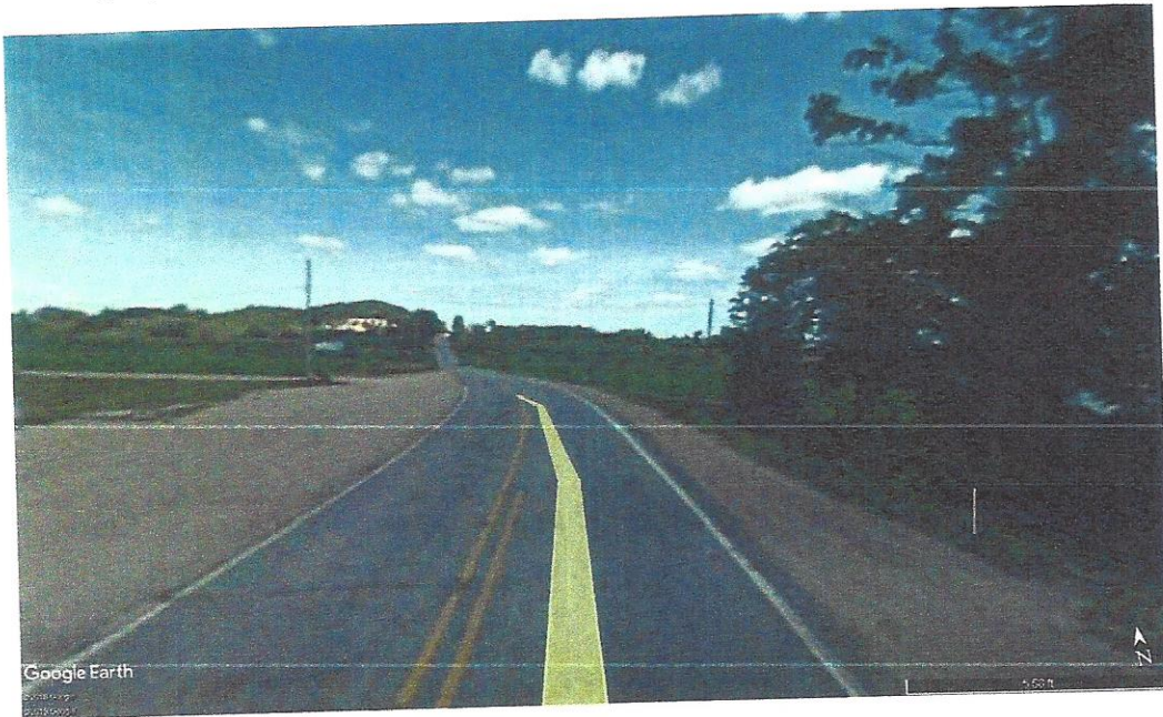
Figure 3 Looking north on 144 th Avenue.
